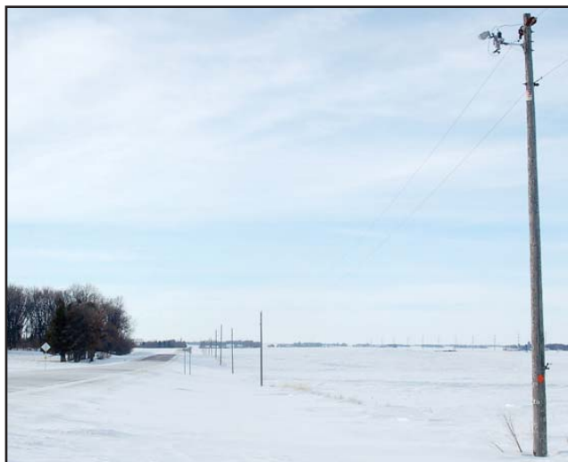
This stretch of overhead line south of Lakefield (along County Road 12) will be changed to underground line in 2023 so a new transmission line can serve a wind farm development.
