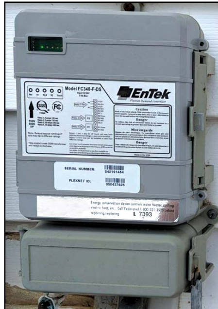
The gray radio control on the side of your house "talks" to your water heater, cooling system or electric heat, if enrolled in one of the co-op's money-saving programs. A green light means it has power. A red light means control is occurring.
