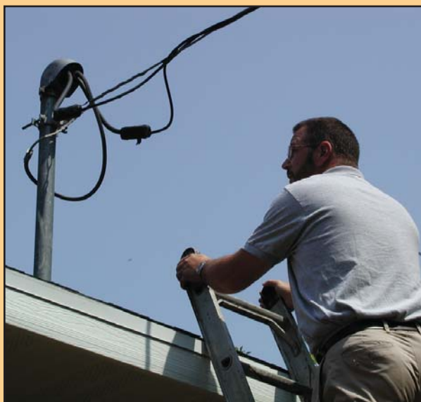
Yikes! Too close! Keep a ladder 10 feet away from power lines, including the connection to your home.
