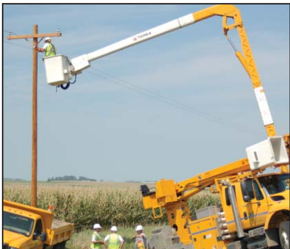
(Above) Nearly done at Dunnell, contractor Highline Construction adds a transformer to this line upgrade in June. Overhead and underground contractors helped out with Federated’s workload rebuilding or upgrading 15 miles of line in both counties.
