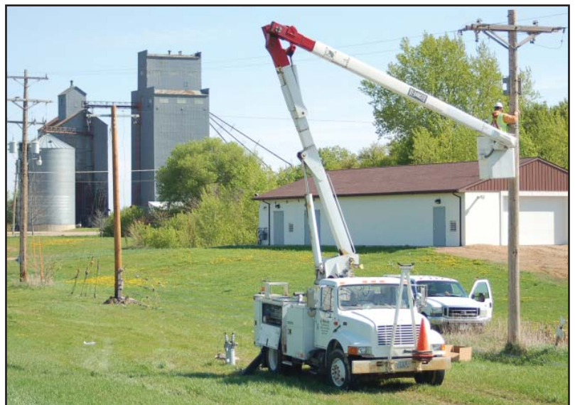
(Above) Nearly done at Dunnell, contractor Highline Construction adds a transformer to this line upgrade in June. Overhead and underground contractors helped out with Federated’s workload rebuilding or upgrading 15 miles of line in both counties.
